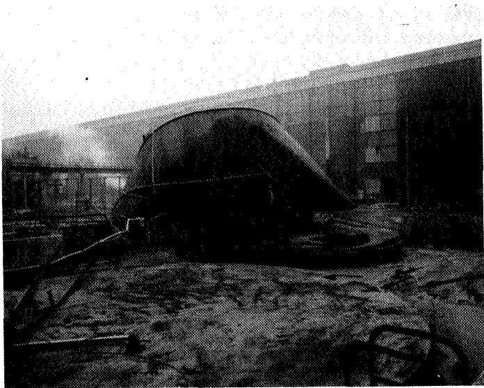
Figure 4. General view across banded area, looking southwest.
